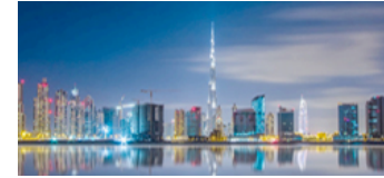
WHERE TO BUILD
