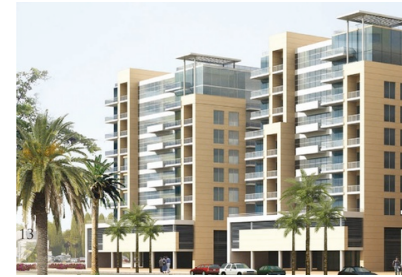
Building: Queue Point Status: Under Construction
